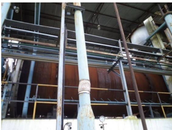
Fig. 7.15 Close up view of a rotary kiln
