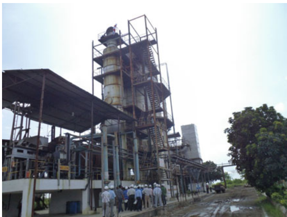
Fig. 7.14 Hazardous waste incinerator
