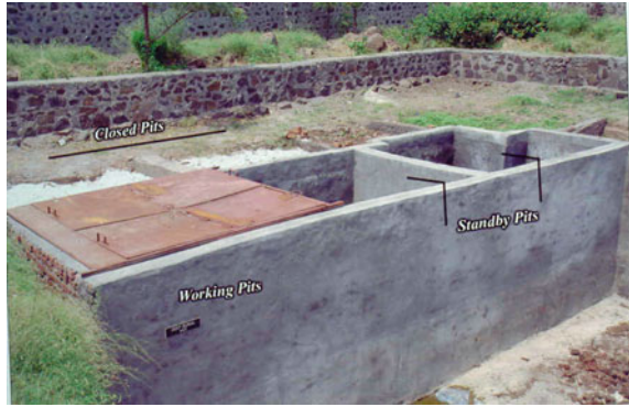
Fig. 6.15 Biomedical waste deep burial facility
