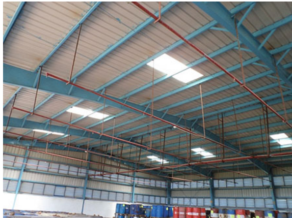
Fig. 11.12 Sprinkler system in hazardous waste TSDF
