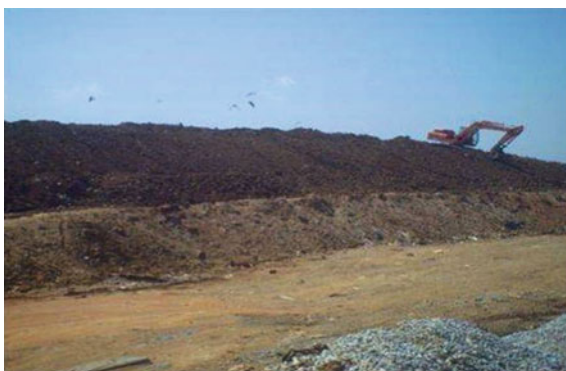
Fig. 5.13 Layering of cover soil on landfill
