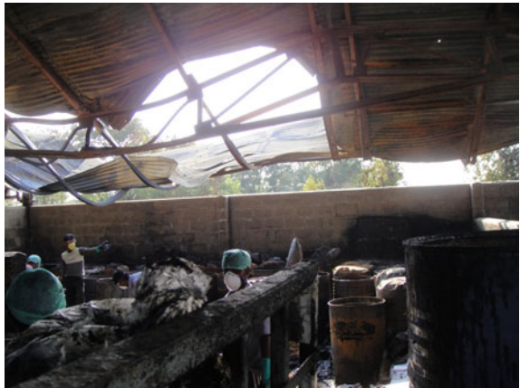
Fig. 13.15 Partially damaged structure during a fire accident
