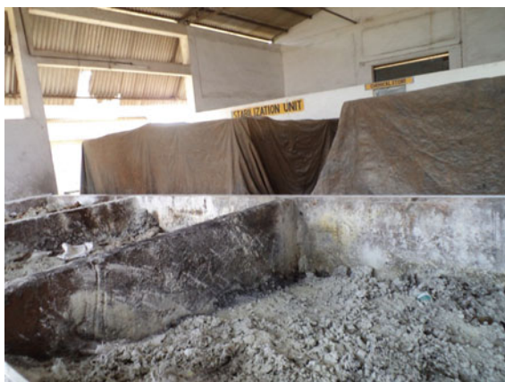
Fig. 7.12 Mixing platforms at a TSDF site
